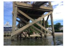
Next we replaced four pile cap's and eight bracing units. We then reconnected the water and electric utilities to all floating docks. Lastly we strengthened the bolted timber connection to the aluminum ramp which lead to the clubs floating platforms.
